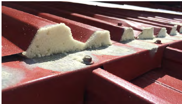
* Silicone on all foam & over joints
