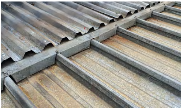
* Silicone 'down slope' & well sealed
