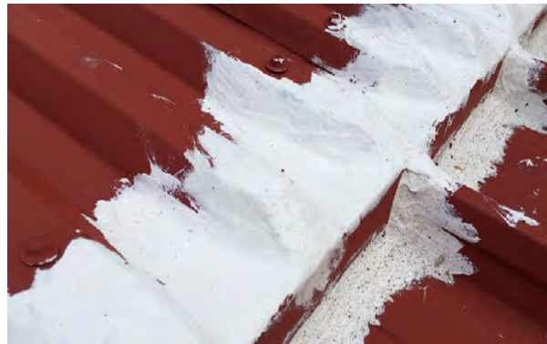
* Silicone applied over join & smoothed
