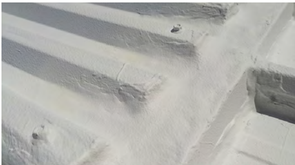
* Silicone 'down slope' & well sealed
