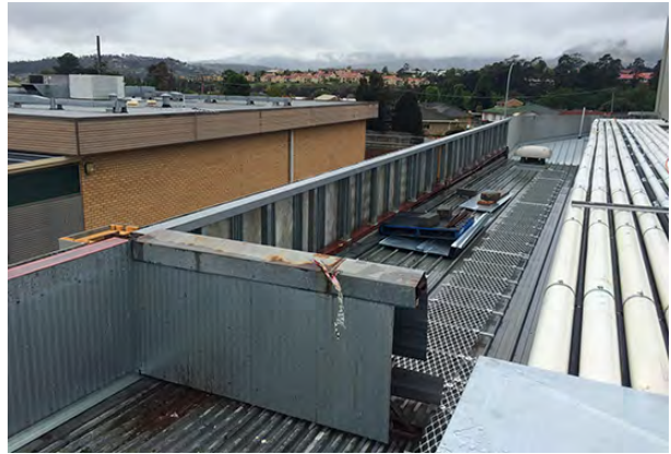
* No capping had been installed
