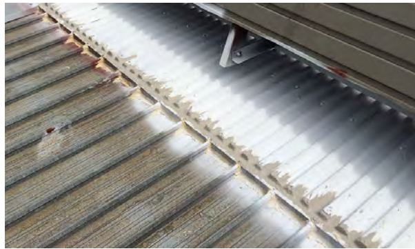
* Silicone on all foam & over joints
