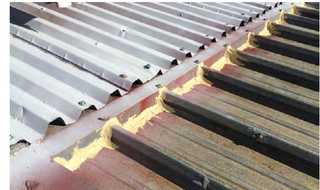
* Closer up view of cut foam
