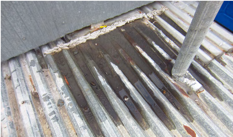
* 'Before' – a horrendous attempt at waterproofing
