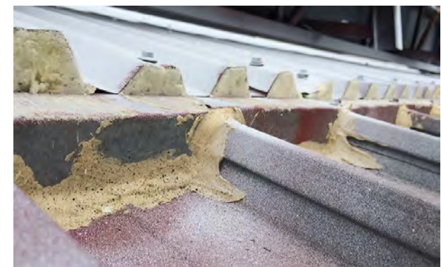
* Closer up view of cut foam
