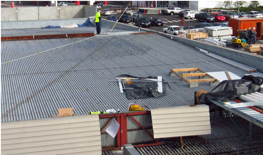
* 'During' – taken during stage 1 power washing
