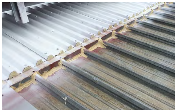
* All external foam cut back off
