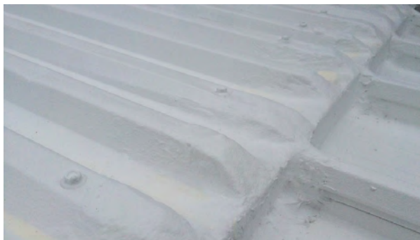
* Silicone almost impossible to spot in areas
