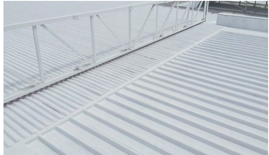
* 'After' – completed waterproofing & coating system:
