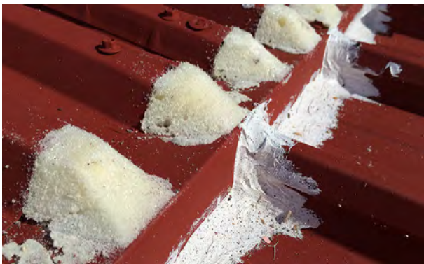
* Foam cut to edge of flashing
