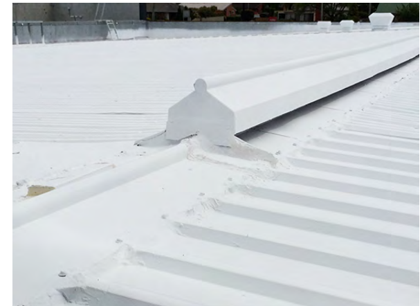
* 'After' – full coating system completed
