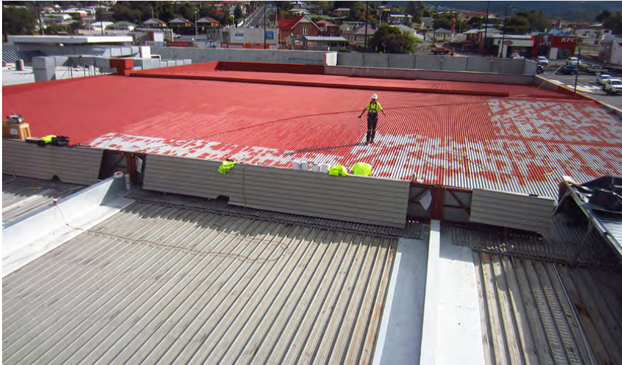
* 'During' – after rust conversion, during rust inhibitor primer
