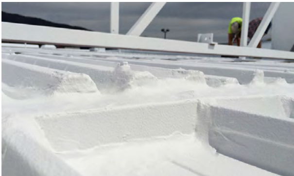
* Silicone 'down slope' & well sealed
