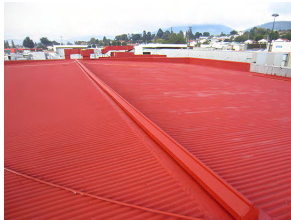
* 'During' – rust conversion & primer coats
