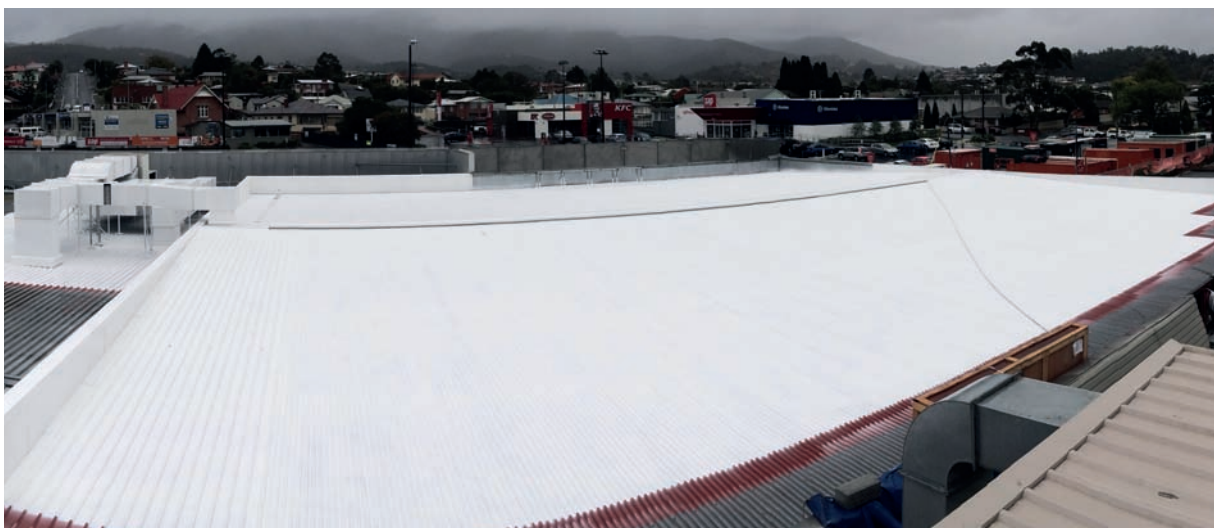
First coat of Thermoshield being applied.
