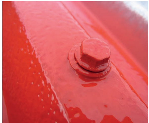
Detail showing the rust conversion, also waterproofing of flashing.
