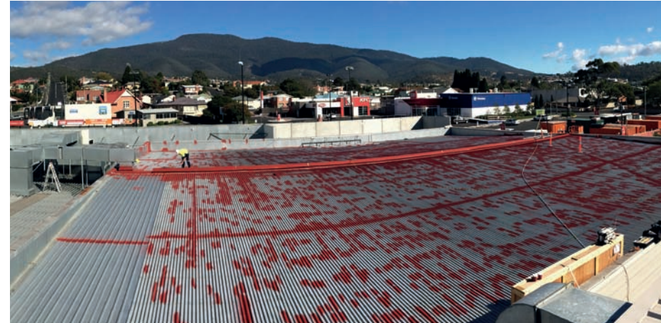
2 – RUST CONVERSION – Applied only to rusted metal
