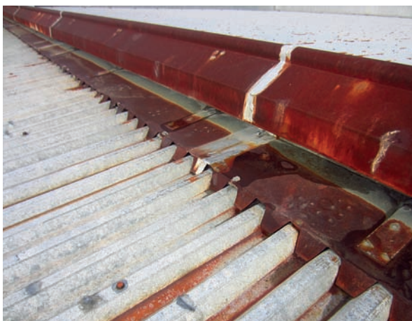
This shows the advanced corrosion of the ridge cap and also the gaping holes where wind can easily push water back underneath, due to the flat pitch.
