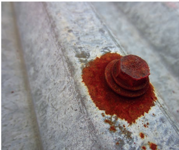
Detail showing the rust conversion, also waterproofing of flashing.
