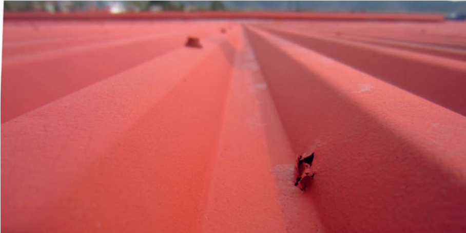
All corrosion holes treated & sealed.
