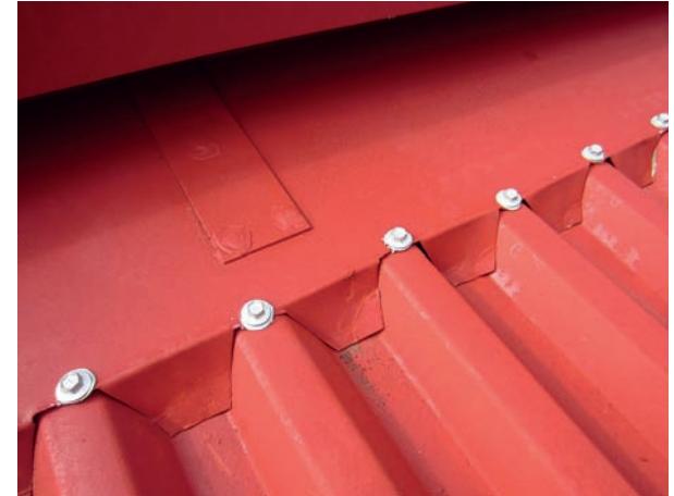
Screw 'down' flashing to sheets.
