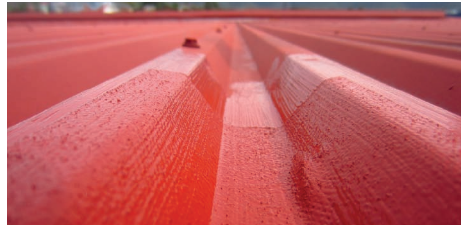
Following rust conversion and prior to the Thermoshield membrane, all non structural holes were repaired and waterproofed.
