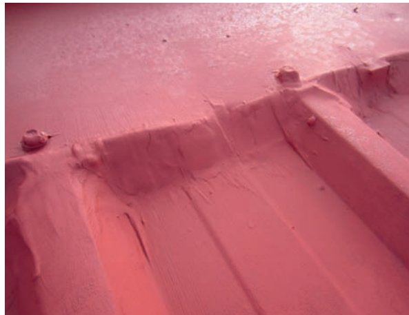
Rust inhibitor etch primer coat.
