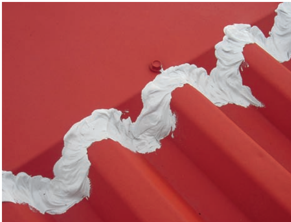
'Gaps' sealed using paintable silicone.
