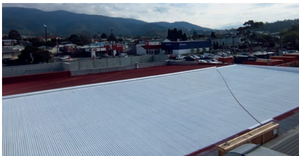
Thermoshield first coat being applied
