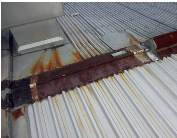
Here you can see on close inspection the zincalume ridge cap is suffering from advanced surface rusting due to the incompatibility between the 'galv' sheeting.
