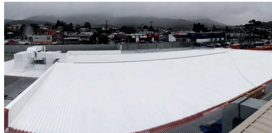
4 – THERMOSHIELD – Thermal ceramic coating applied
