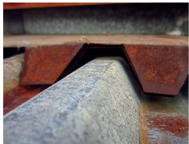
This shows the advanced corrosion of the ridge cap and also the gaping holes where wind can easily push water back underneath, due to the flat pitch.
