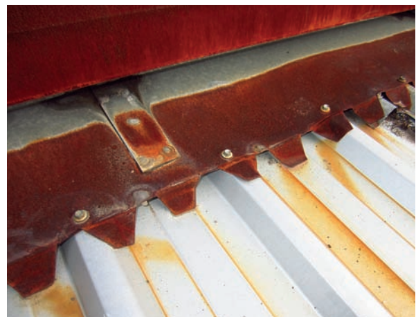
Here you can see on close inspection the zincalume ridge cap is suffering from advanced surface rusting due to the incompatibility between the 'galv' sheeting.
