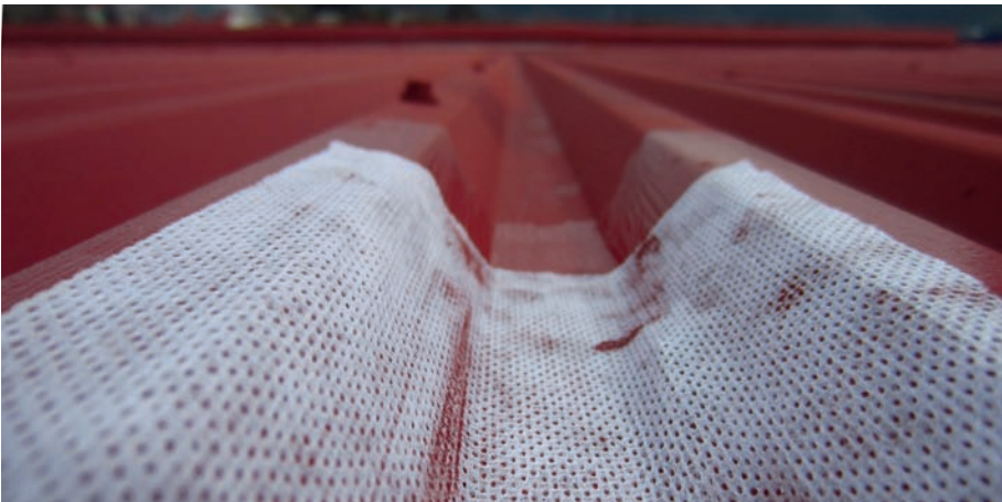
Following rust conversion and prior to the Thermoshield membrane, all non structural holes were repaired and waterproofed.
