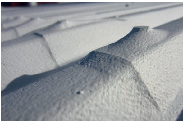
First coat of Thermoshield being applied.
