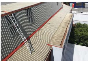
Water pooling around penetrations caused surface rusting:
