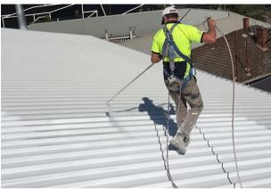
Contrast between white first coat and shale grey second coat:
