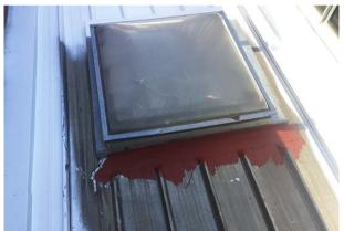
Most flashings were/are galvanised steel whereas the roof sheeting is zincalume. The electrical mismatch in the dissimilar metals resulting in accelerated corrosion of the flashings:
