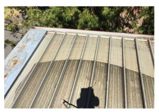
In addition to the roof sheets, gutters that were completely filled with debris were cleaned and power washed:
