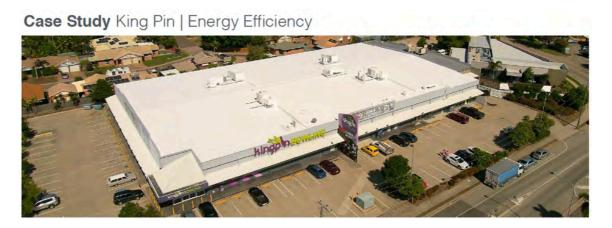
Project location is Townsville QLD. This example is ideal due to Townsville having year round heat & solar radiation exposure. Strongly demonstrating HVAC reduction due to the Thermoshield coating & BMS installation allowing for a more tailored and reduced energy setting profile.
