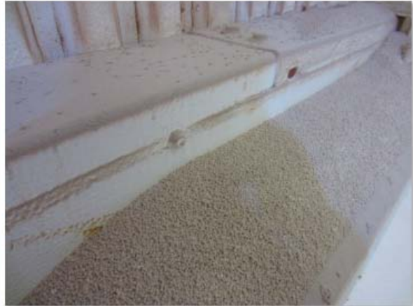
* Bay 2 - sheet joins & screws sealed. Piled AN 'harmless'
