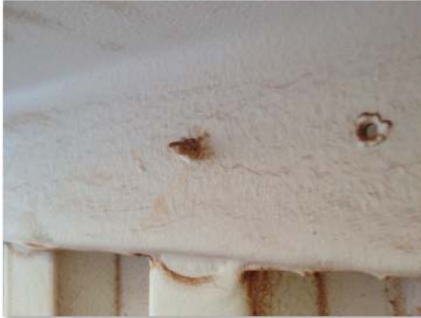
* Close up internal purlin penetrations - heavily sealed
