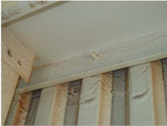
* Purlins 'flooded' - where tech screws had entered
