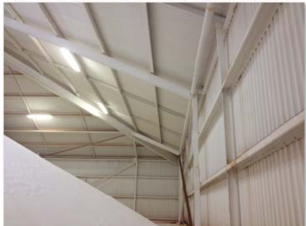
* Internal coating shed 1 (east) wall - no visible corrosion
