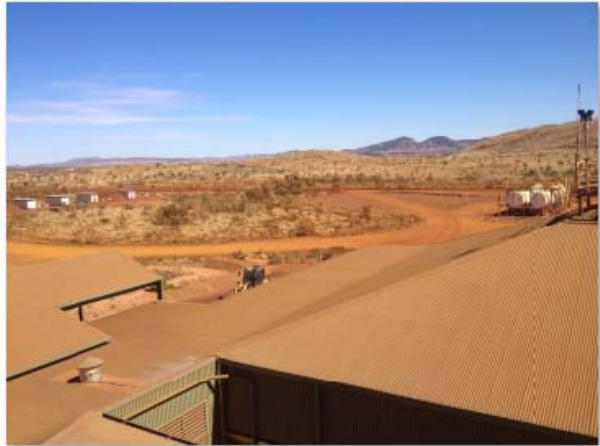
*Shed 2 roof & front apren - no visible corrosion
