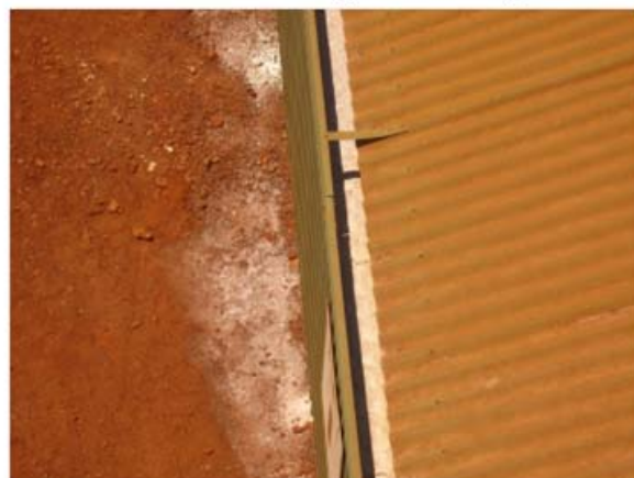
* AN has ran down the sheeting - to collect in gutters
