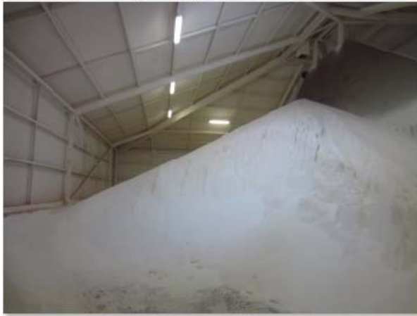
* Shed 1 (west bay) - no signs of corrosion
