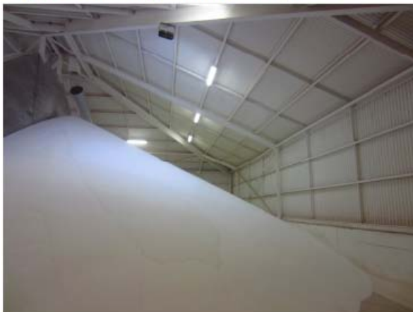
* Bay 1, shed 1 - no signs of corrosion or product failure
