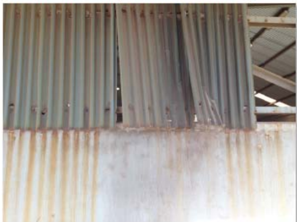
*Internal wall sheeting - imminent risk of falling
