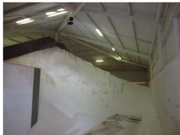
* Bay 4, shed 3 - no signs of corrosion or product failure
