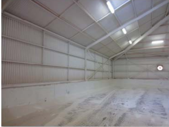
* Bay 2, shed 1 - no signs of corrosion or product failure
