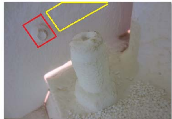
*Sheet joins, penetrations & screw/bolt thread sealed
