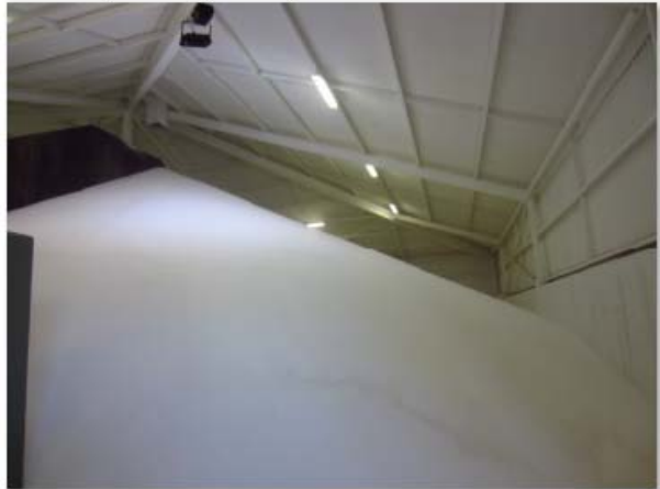
* Shed 2 (east bay) - no signs of corrosion
