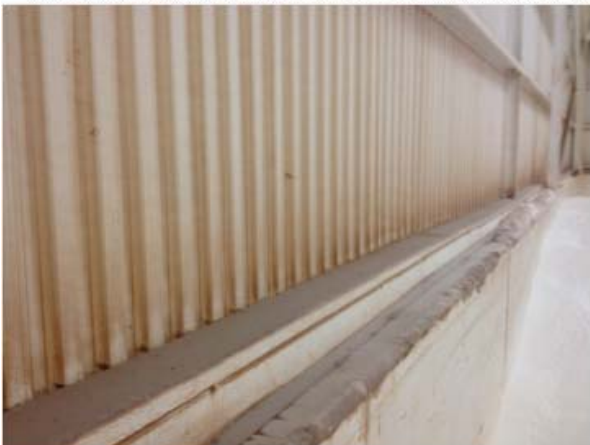
* Internal coating shed 1 (west) wall - no visible corrosion
