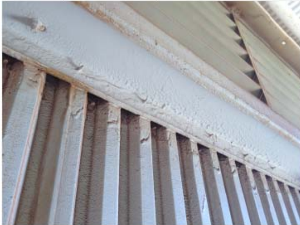
* Wider angle internal coating - no visible corrosion
