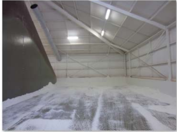
* Shed 1 (east bay) - no signs of corrosion
