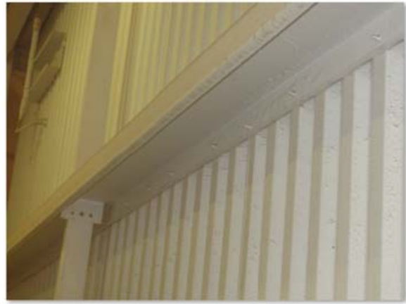
* Tech screws touched up by hand to ensure 'seal'
