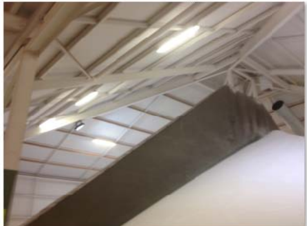
* Internal roof coating - no visible signs of corrosion
