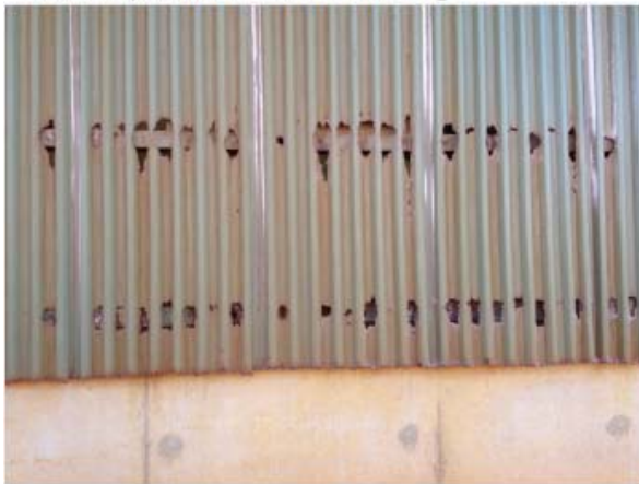
*Roof sheeting corroded in corrugation 'troughs'
