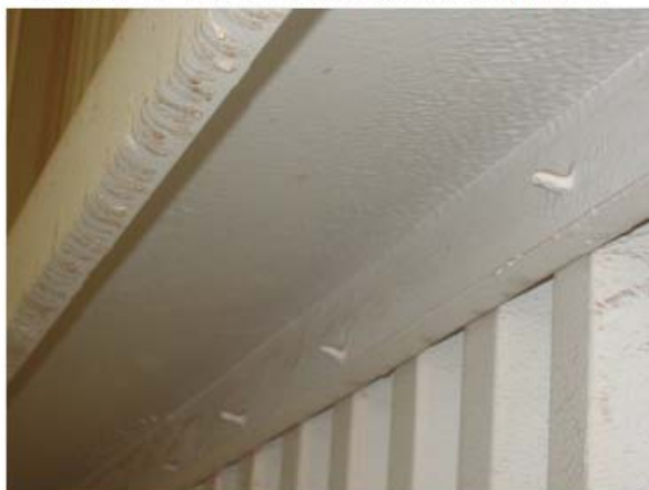
* Bay 4, shed 2 - penetrations in purlins heavily sealed
