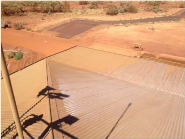
*Shed 1 roof - no visible corrosion
