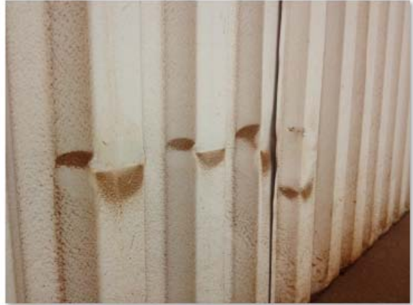
* Flexible coating undamaged - despite major knock
