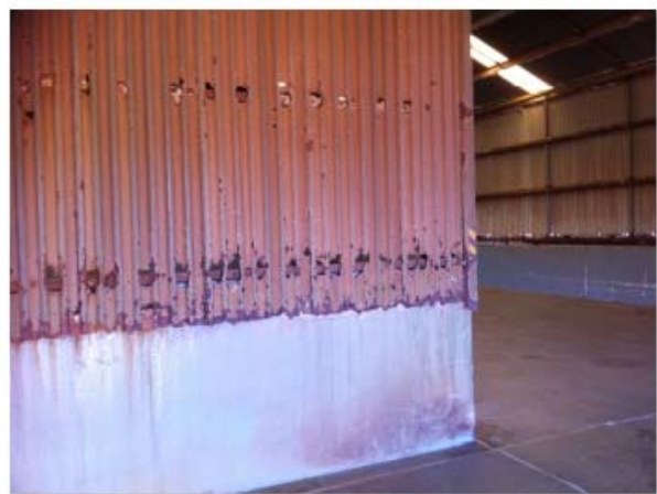
*Replaced sheets in bay 1 - with 'protective' coating
