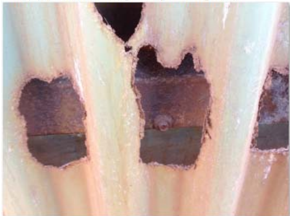
*Internal wall sheeting - imminent risk of falling
