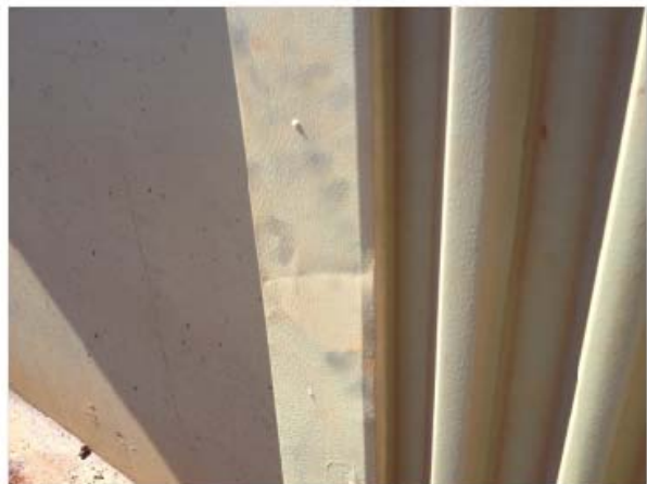
* Flexible membrane has withstood many knocks/bumps
