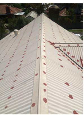
The 'polka dot' contrast of the roof sheet to rust converter highlights how widespread corrosion & rust rusting had become underneath the moss & mould coverage:
