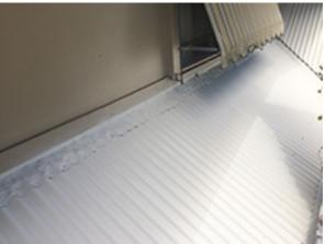
You can see from the below photo how the tech screws have been well sealed beneath the ceramic coating. If the problematic screws are not able to come into contact with water or oxygen, then they are deprived of essential elements to cause further corrosion.
