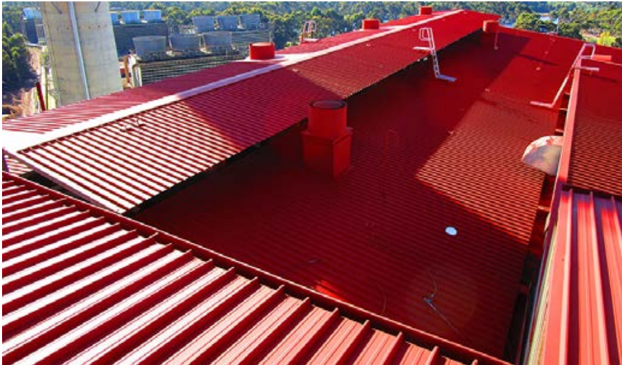
Rust inhibitor etch primer applied:
