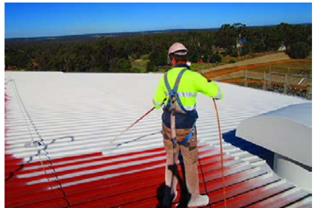
Forehand pass – completing front side of rib:
