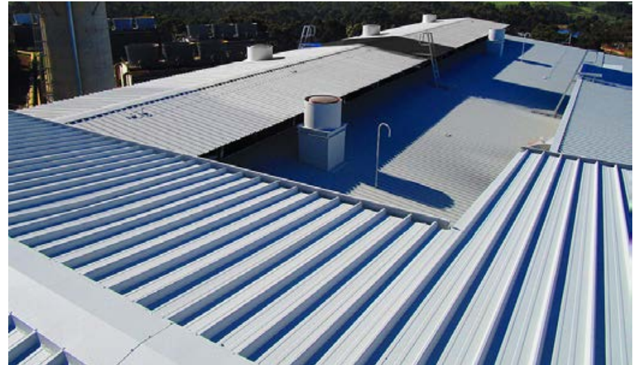
3 x Thermoshield coats | Completed coating system:
