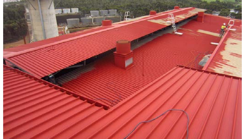
3 x Thermoshield coats | Completed coating system:
