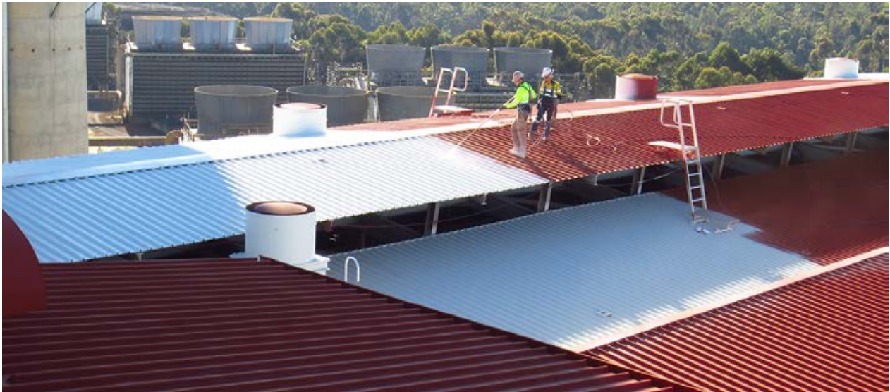
Backhand pass – focusing on reverse side of rib:
