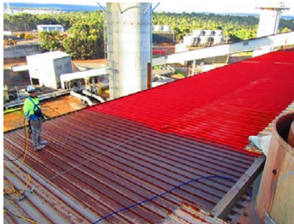
Rust converter being applied:
