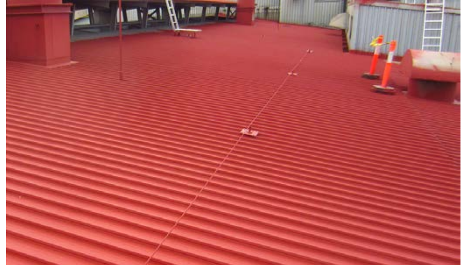
3 x Thermoshield coats | Completed coating system:
