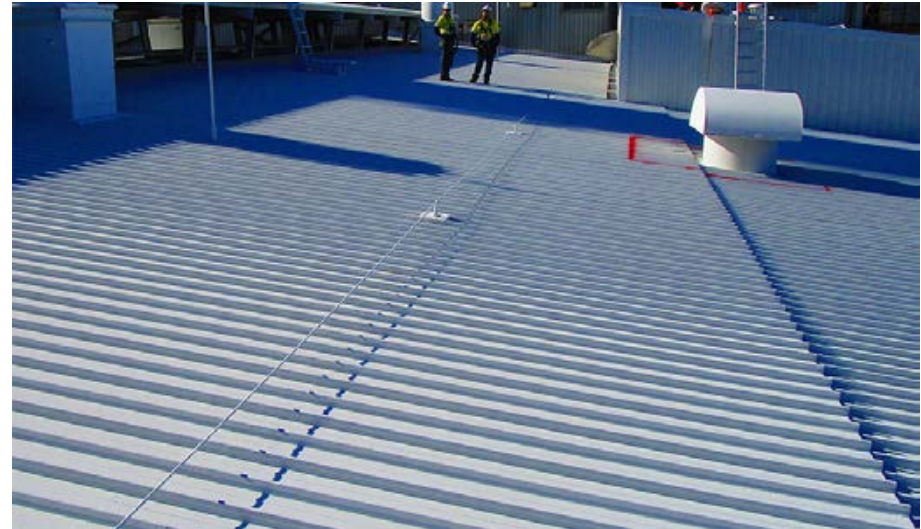
3 x Thermoshield coats | Completed coating system:
