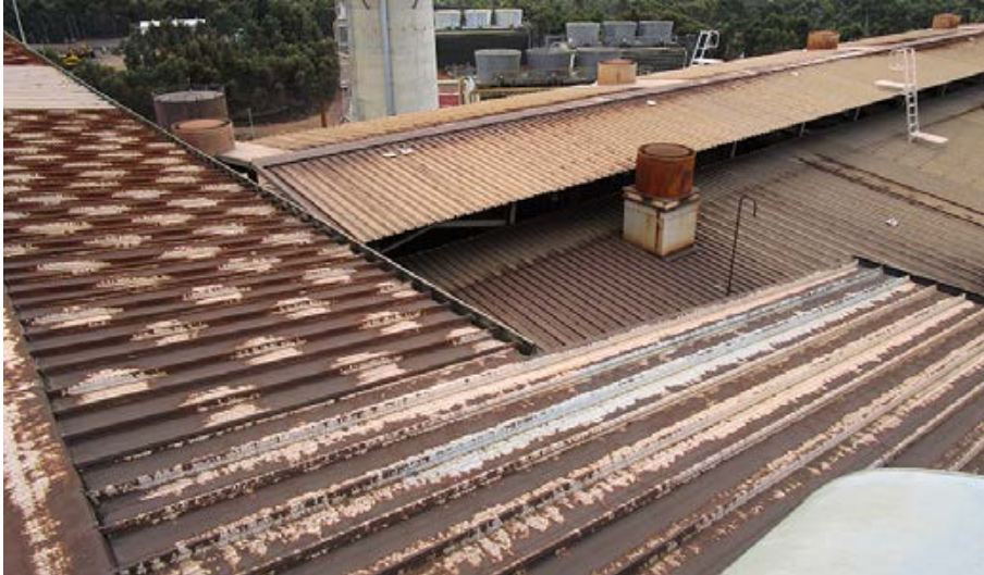
Rust inhibitor etch primer applied:
