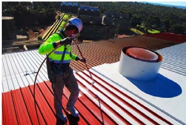
Backhand pass – focusing on reverse side of rib:
