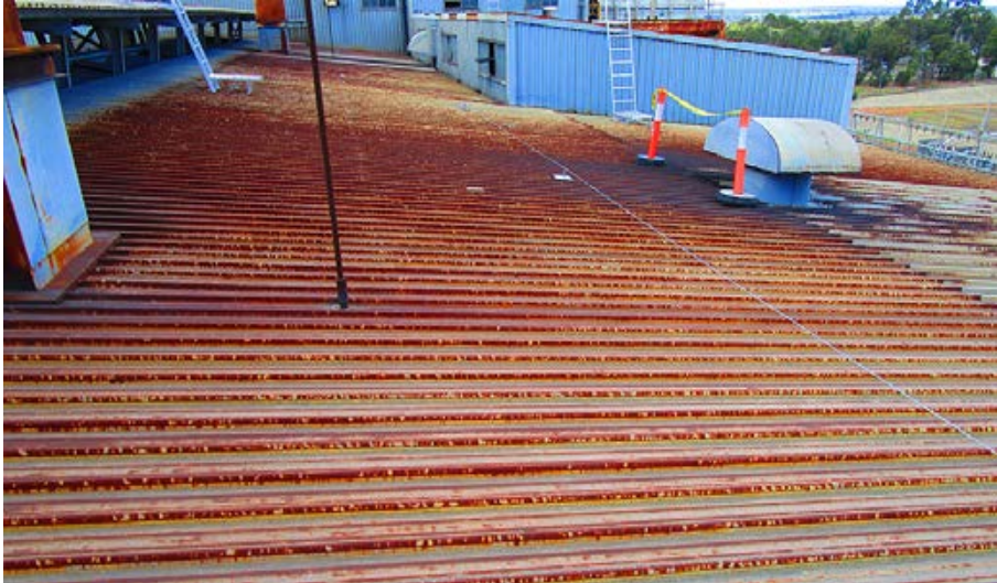
Rust inhibitor etch primer applied:
