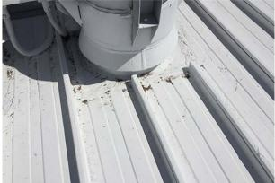
Below photos show the comprehensive sealing of sheet overlap and tech screw penetrations:
