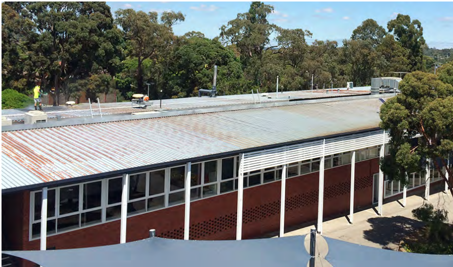
* DURING – Second coat (shale grey over white)
