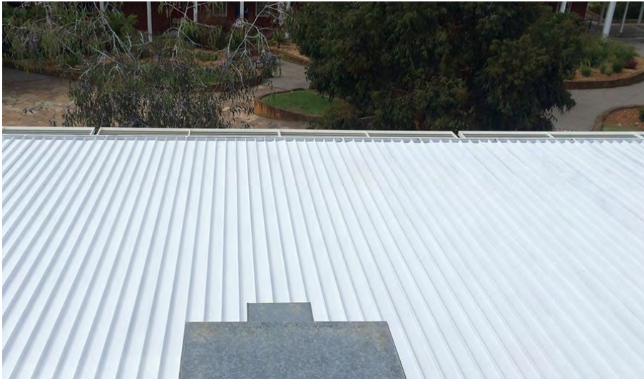
* DURING – First coat (White Thermoshield)
