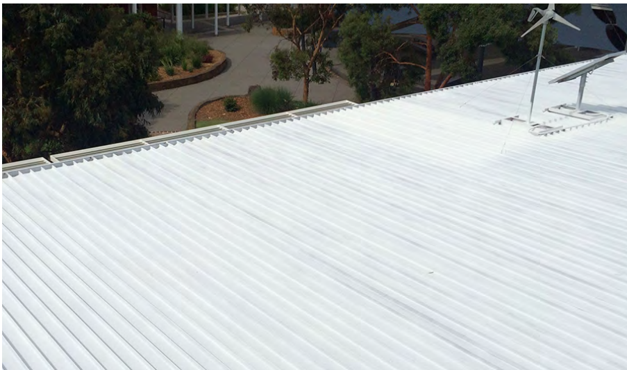
* DURING – First coat (White Thermoshield)
