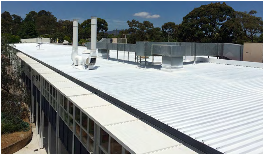
* DURING – First coat (White Thermoshield over rust converter)
