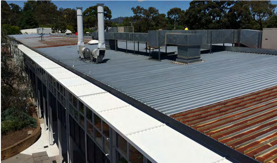
* DURING – First coat (White Thermoshield over rust converter)
