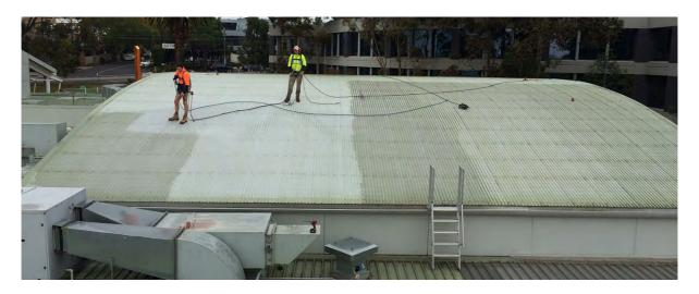
Power washing from static line & harness – rope set to safe length to avoid fall:
