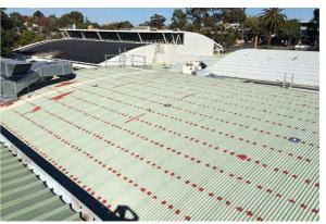
New anchor points were masked up & in addition, old anchor points & sheet joins were heavily waterproofed:
