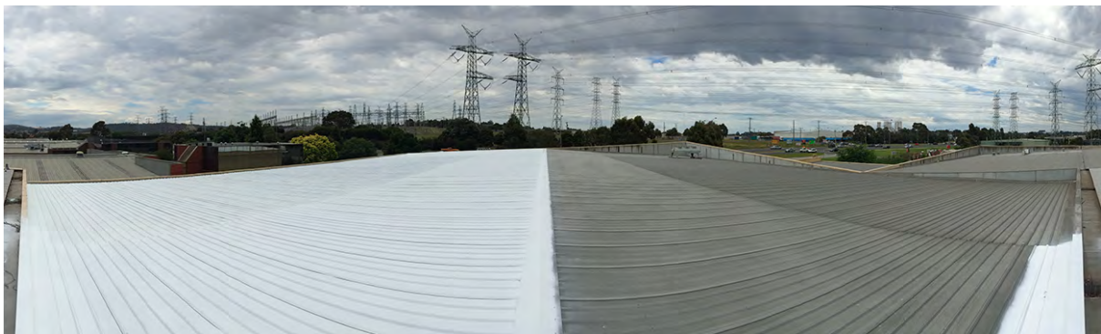
Finished coating (2 x 500micron coats of Thermoshield):
