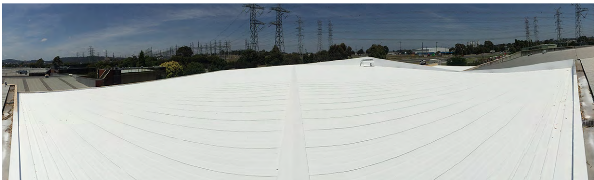
Finished coating (2 x 500micron coats of Thermoshield):
