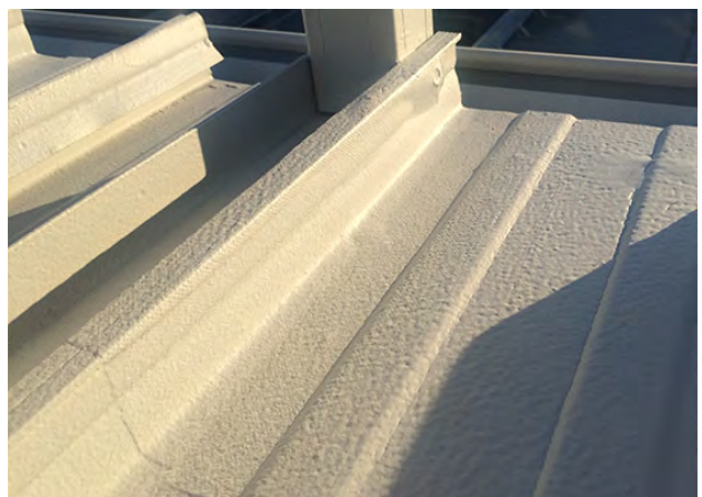
Step 5: Sealed beneath TS coating [shale grey]
