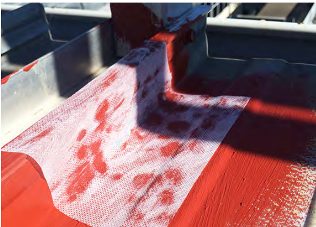
Step 4: Sealed beneath TS coating [white]
