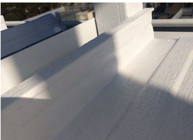
Step 4: Sealed beneath TS coating [white]
