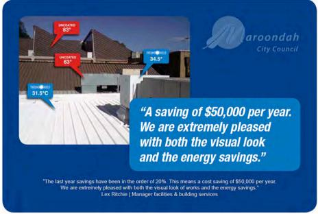
Above [right] shows a progress photo whereby temperatures were recorded to compare the difference between the uncoated metal.
