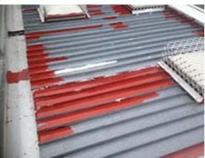
Below are additional photos showing the cleanliness of the roof sheeting which ensures maximum coating contact — also shown is the care taken to apply rust conversion by hand:
