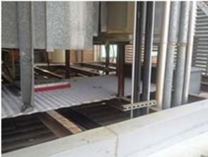
You can see from the below photo how the roof was covered heavily in dirt and oil & grease – which is a certain precursor for corrosion:
