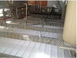
The above & below photos demonstrate the comprehensiveness of the coverage. When coating a roof with a relatively steep pitch – each coat is applied focusing on a particular direction, meaning there may be areas of "shadow". However on the subsequent coats, the angle of approach is reversed and any shadows are well sealed.
