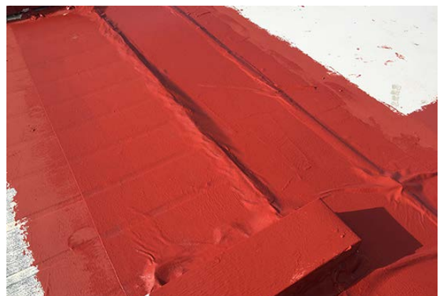
Bridging the old/new roof join:
