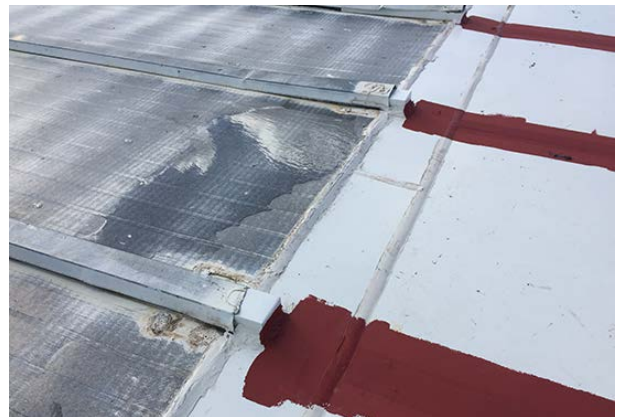
Bridging the old/new roof join:
