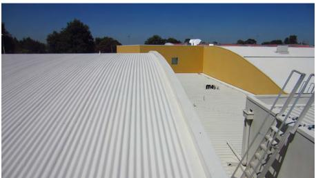
The primary purpose for the Thermoshield restoration was for rust conversion & providing a protective membrane to prolong the lifespan of the roof. In addition, the roof has come up like new, replacing the tired & faded appearance.
